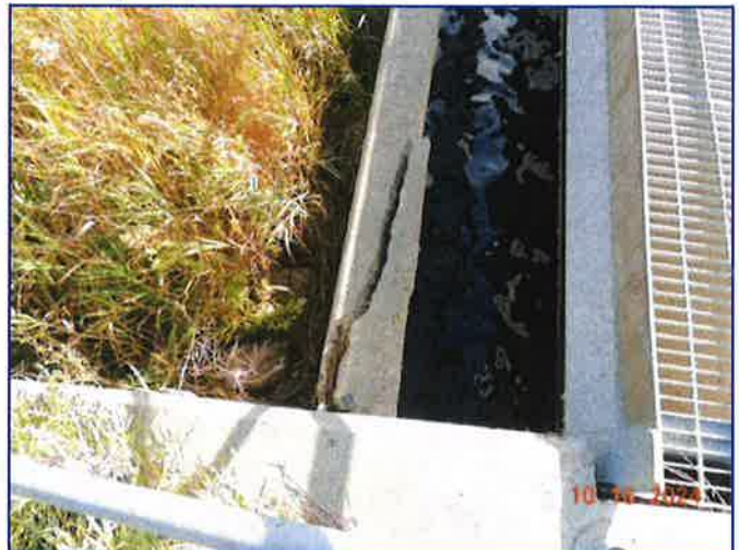
Photo 10 (lower right) - Another view of the crack in the right concrete weir at the abutment wall.
