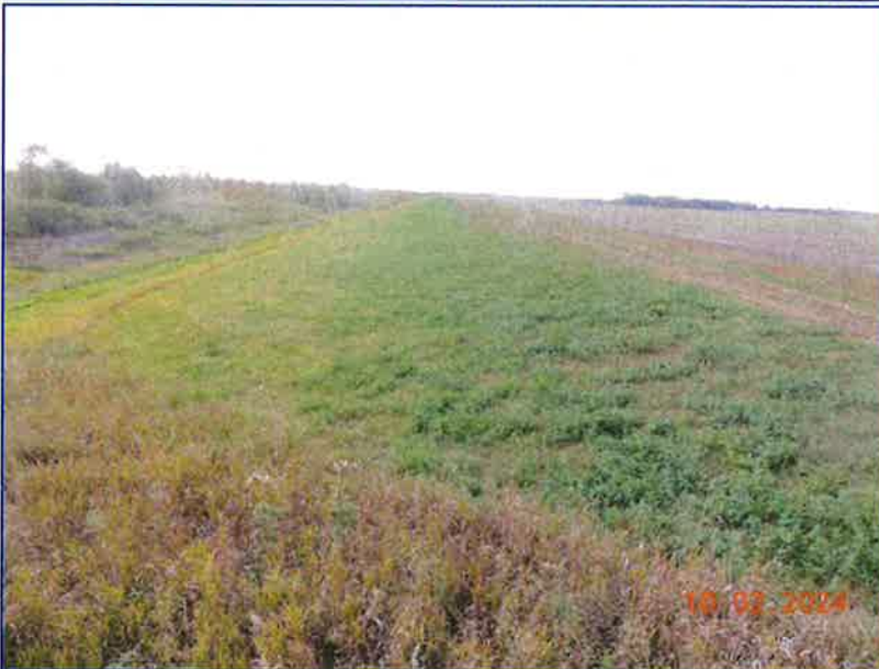
Photo 8 - The earthen embankment is in good condition and nicely maintained.
