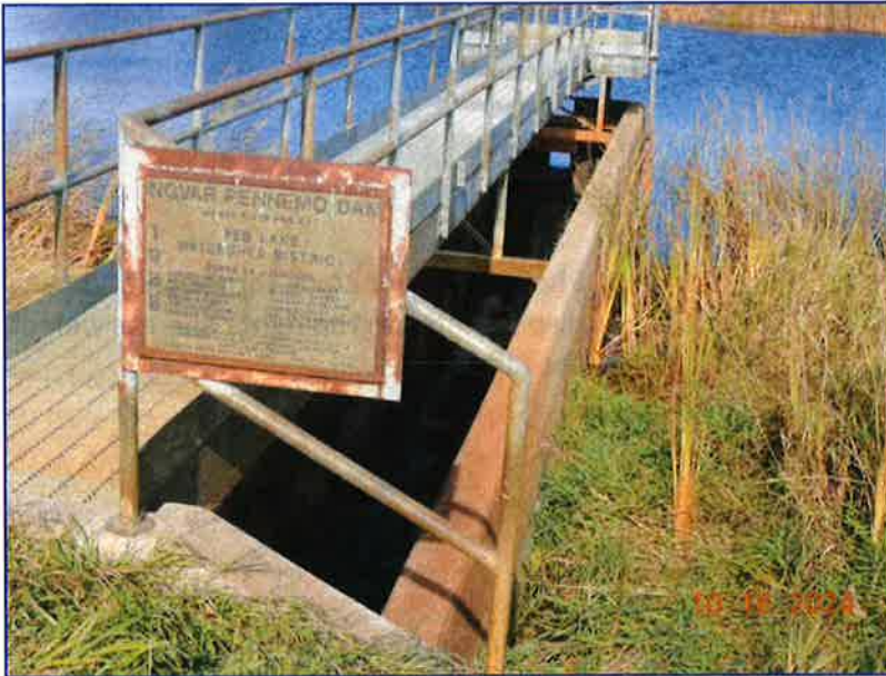
Photo 11 - Left concrete weir and walkway for the southern outlet structure.
