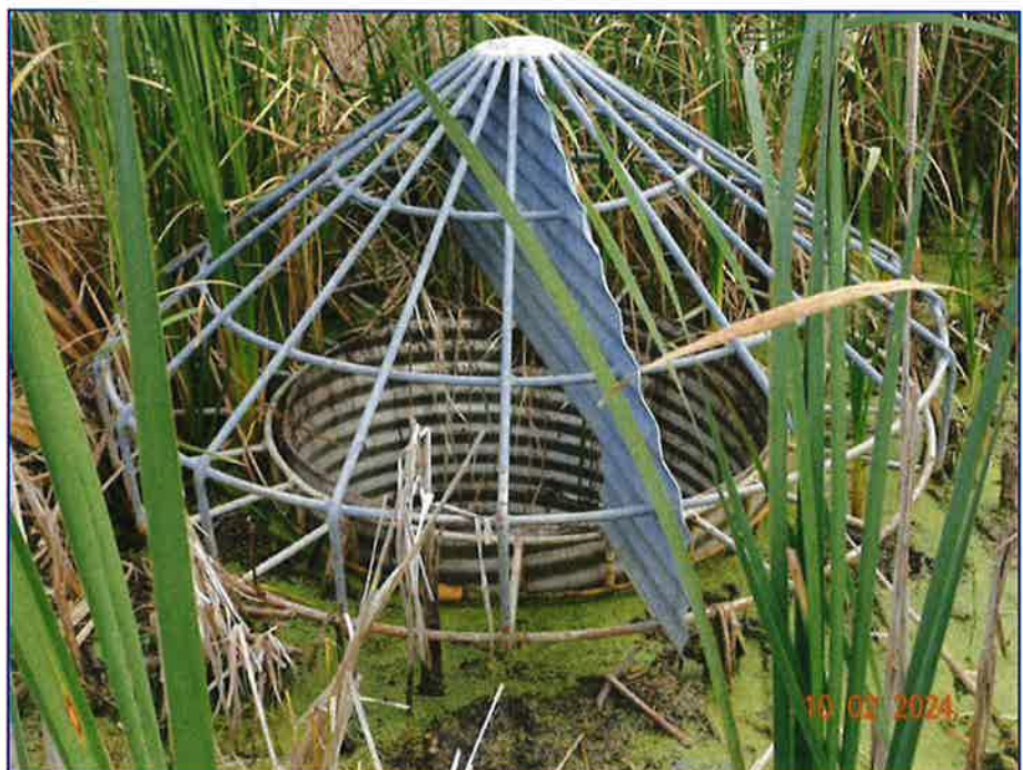
Photo 2 - Vegetation around the riser inlet.
