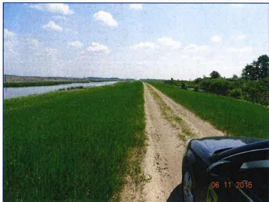
Photo 2 - Typical embankment and crest road. Photo from 2015.
