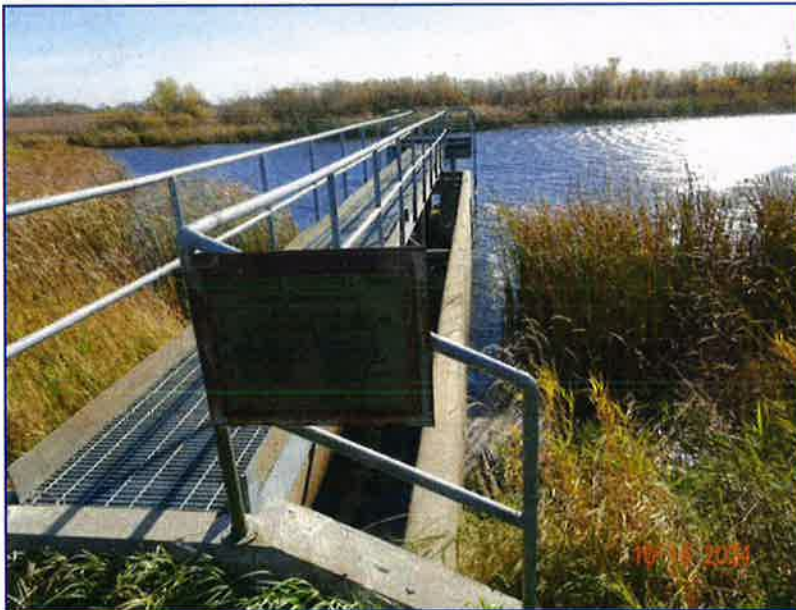
Photo 4 - A Walkway and left concrete weir crest.
