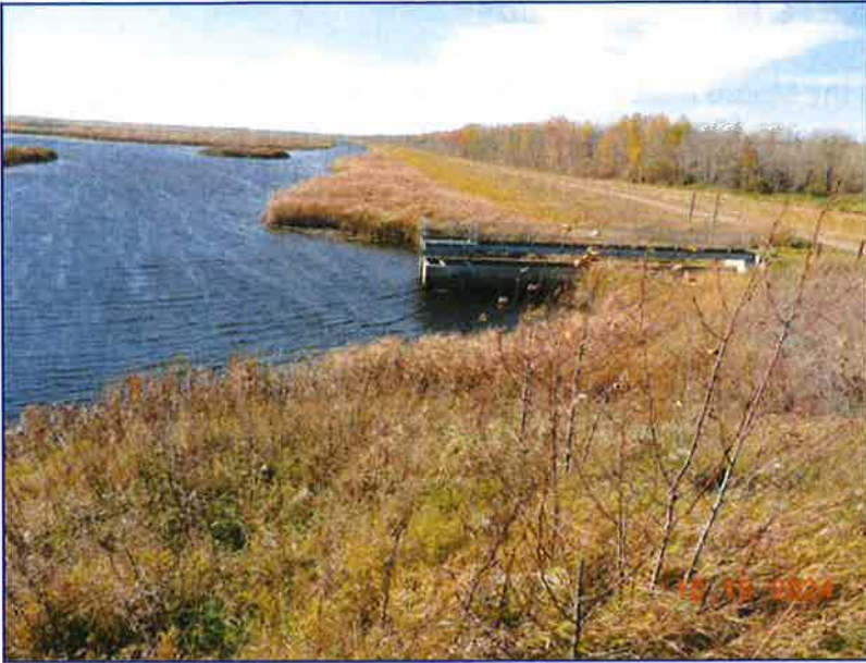
Photo 3 - Overview of the northwest control structure.
