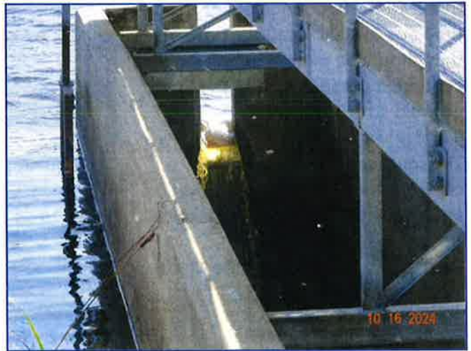
Photo 6 (lower right) - Right weir crest and upstream low flow inlet.
