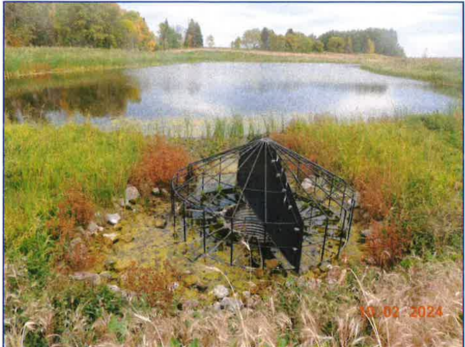
Photo 1 - Thibert Pond and the new riser inlet.
