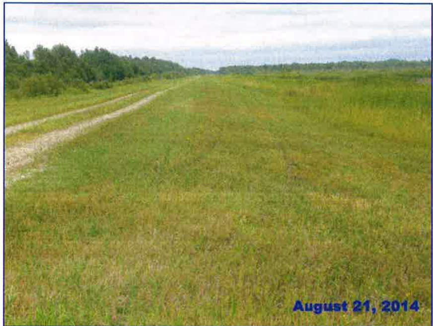
Photo 1 - Typical embankment and crest road. Photo from 2014.
