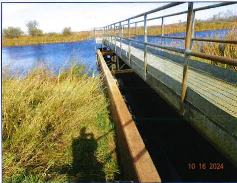
Photo 12 - Right concrete weir for the southern outlet structure.
